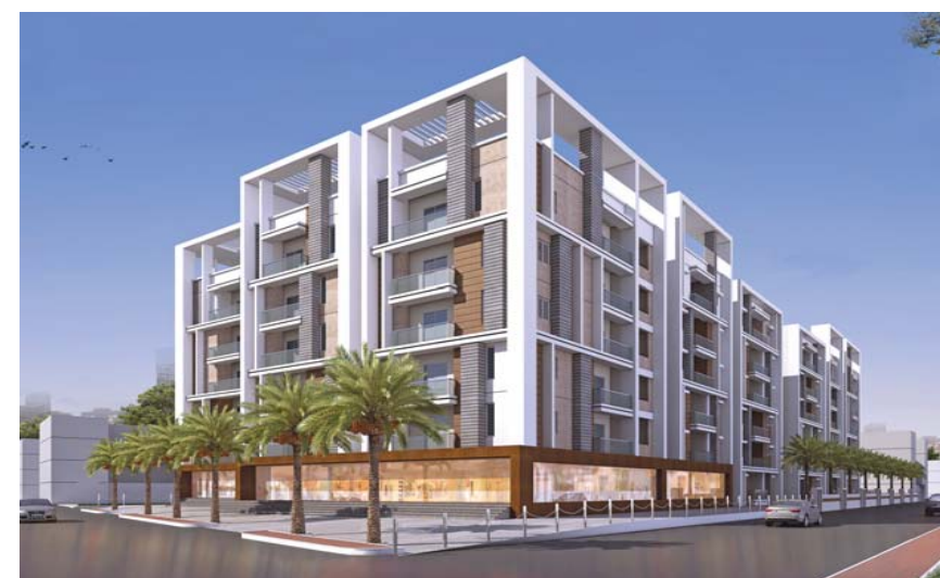
84 Luxury Flats @ Alkapoor Township
